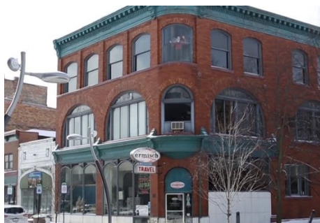
Inge's Place A local business incubator and showcase, offering office space for start-ups, small non-profits, and anyone needing space to get work done.
